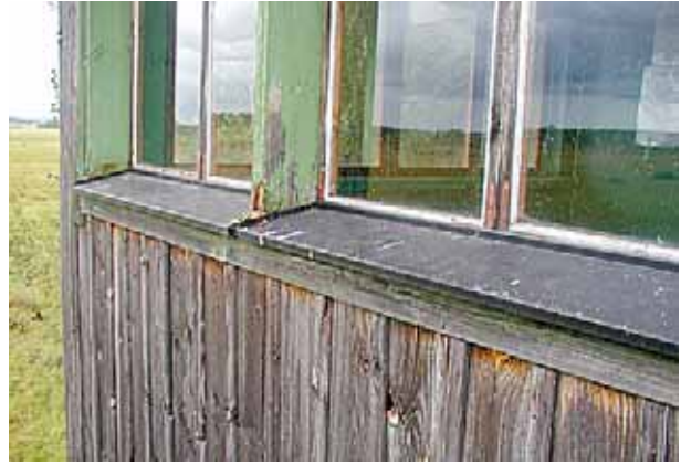
Painted with tight paint has caused rot on windows. Unpainted parts still okay after 50 years!
