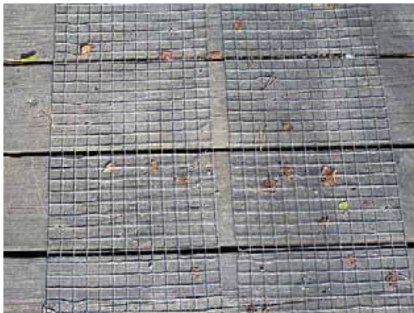
Net of metal on the trail to prevent accidents when it is slippery
