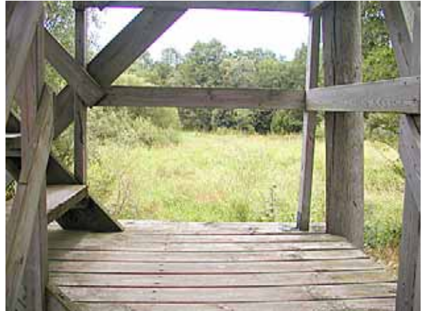
A big opening that children and adults could fall through when falling in the stair.
