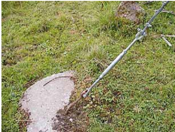
An adjustable wire makes the tower more stable.
