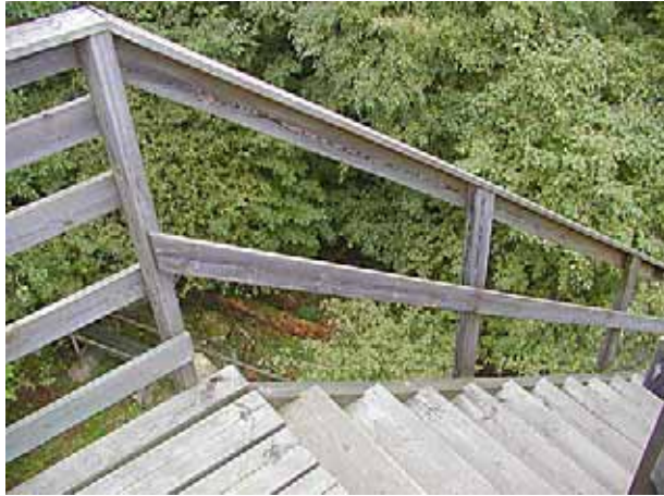
This steep stair constitutes a severe risk in case of a fall. The fact that it is high and has a sparse railing increases the risk.
