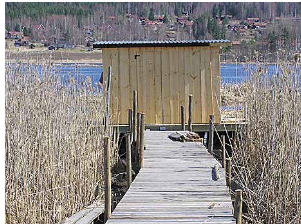
A wide footbridge leading towards a hide under construction. Reliable railings and screens to shield the bridge from birds in the water are waiting to be put up.
