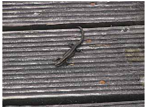
Trail built of planks with tracks on upper side. Gives a less slippery surface.
