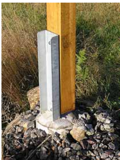
Foundation of a sign stand. A long lasting construction of concrete, but design could maybe be better?
