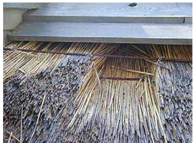
Ducks have picked out the reed straws from this roof. Protection with nets can prevent damages.
