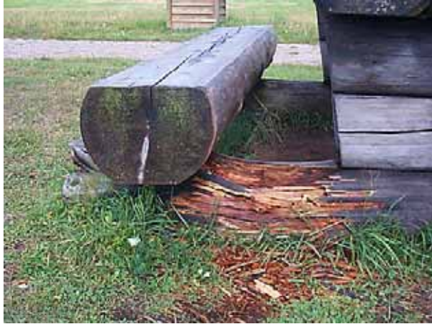
Standing directly on the ground. Starting to rot after just a few years.
