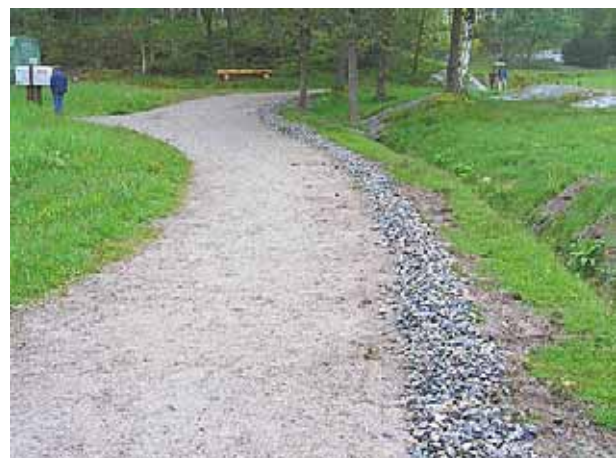
A surface with different colour makes it easier for a person with impaired vision to use the trail.
