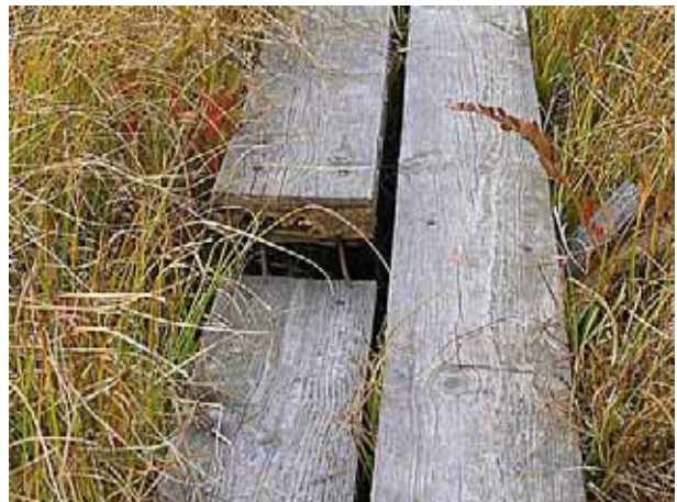
Trail over wet bog. It has started to rot and becoming dangerous. Time to rebuild.
