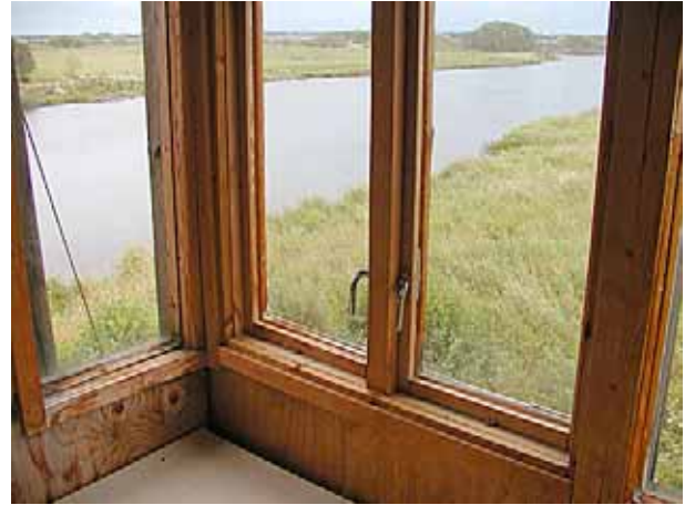
It is easy to get problems with condensation on windows in unheated spaces. Here water has run down the wall.
