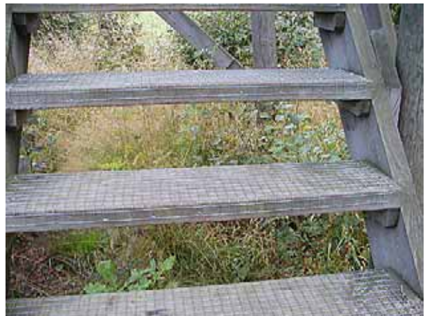
A net has been put in to the far too steep stair, to give a better grip at damp weather.
