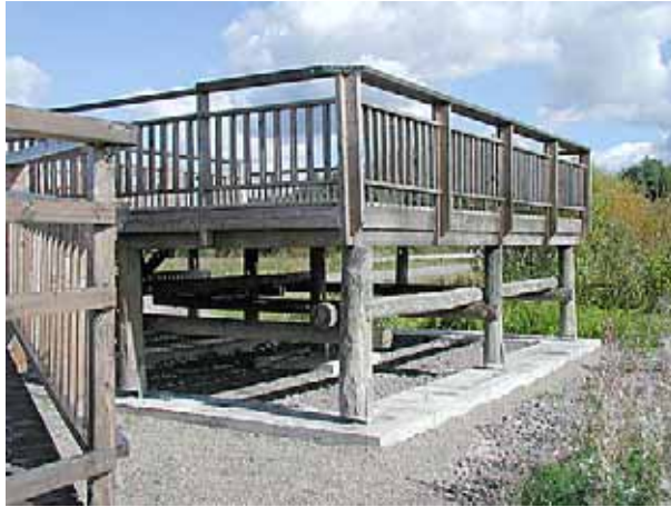
Example of good foundation. Big distance between wood frame and foundation prevents moisture absorbance.
