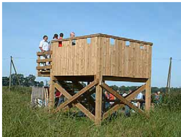
Platform with openings in the rail, making it possible for children to see through the rail. Germany, Delver Turm
