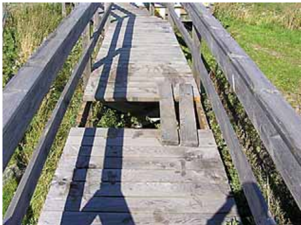
Regular maintenance is important. Not easy to pass this hole with a wheelchair.
