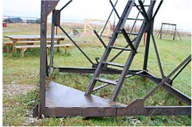
High steep stairs with a narrow step of some steel bars is a big risk for falling accidents.
