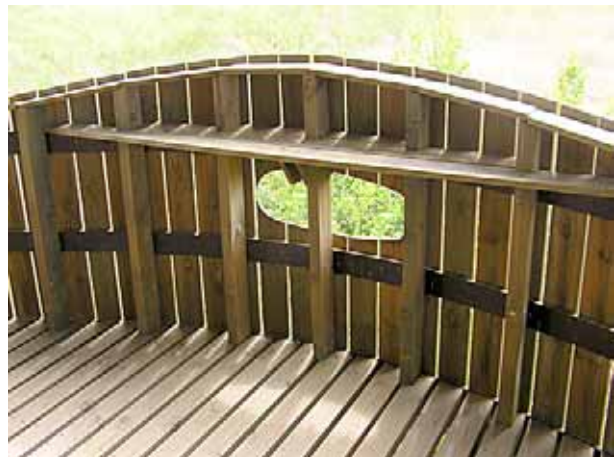
Good example of a rail with smaller openings for children. From security aspects the opening the opening should be a little bit smaller.
