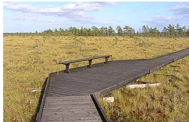
Trail on wet ground built of wood. Expensive to build and maintenance as well.
