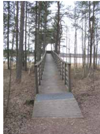
A grating at the start of the ramp reduce the amount of gravel and soil in the tower.
