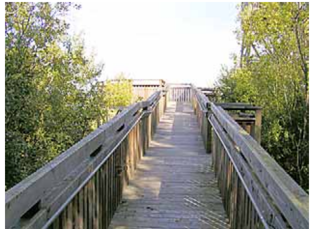
Good example of a ramp, wide enough and with stable railings on both sides. The ramp also contains ledges on regular intervals.
