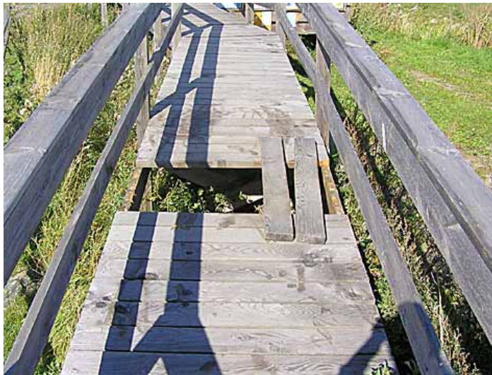
By useing screws can prevent planks from being pulled out.
