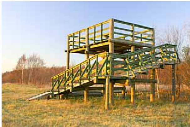
By building a ramp around the tower, steep stairs can be avoided
