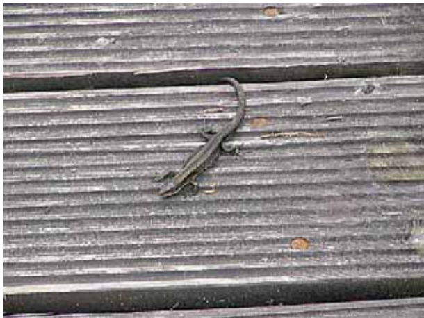
Example of a path assembled with tracked boards to decrease the slipperiness.
