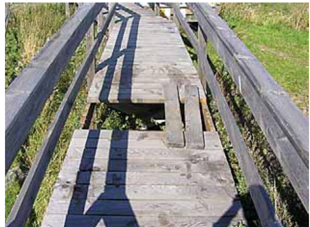
A well designed ramp that has been vandalized. Imidiate repair is required to make it usable for wheelchairs.
