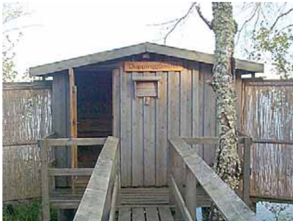
A footbridge leading to a hide, which has been screened of from the birds in front by large screens made of reeds. Proper railings along the footbridge prevent people from falling off. The narrow width however, makes it impossible for most people in wheelchairs to visit the hide.
