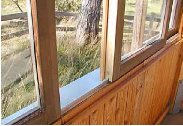
Windows that can be pushed aside to open. Difficult to get tight joints that withstand rain.
