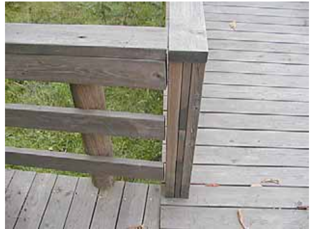
Ramp separated from the platform to prevent vibrations. Here the opening need to be adjusted after subsidence.
