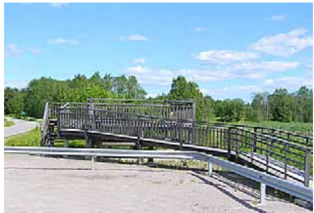
This tower is located in a slope of an embankment, which facilitates the connection of the ramp.
