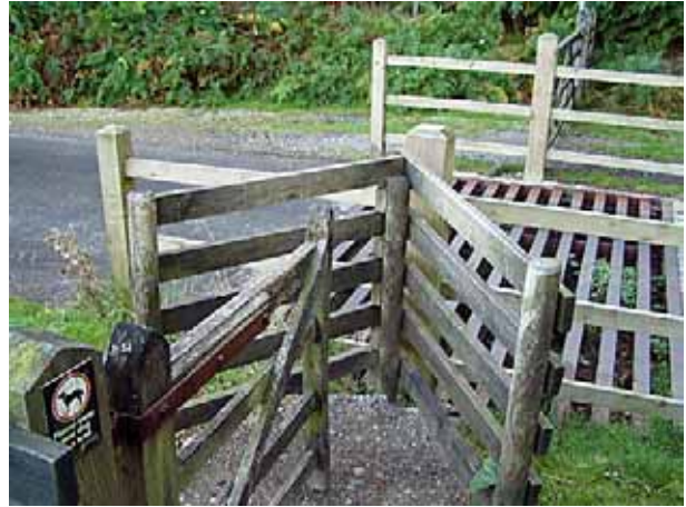
Cattle grid combined with a gate that can be opened.
