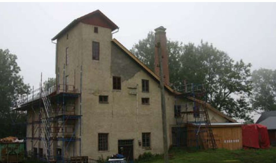
Annebergs bränneri under renovering.
