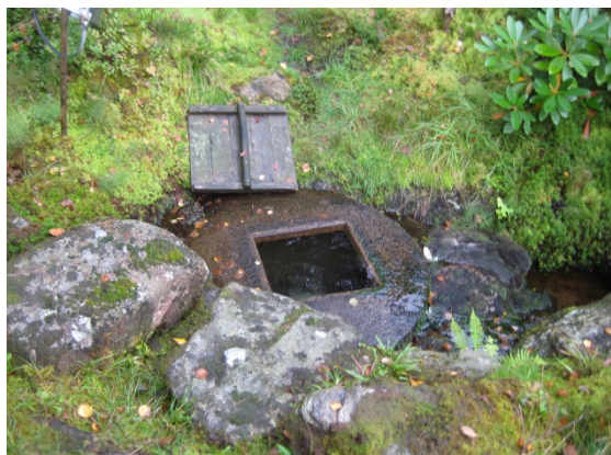
Figur 5 Station 809 Hallen. Brunnen har lock.
