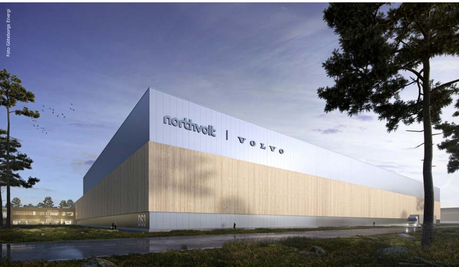
NOVO Energys batterifabrik i Torslanda, Göteborg.
