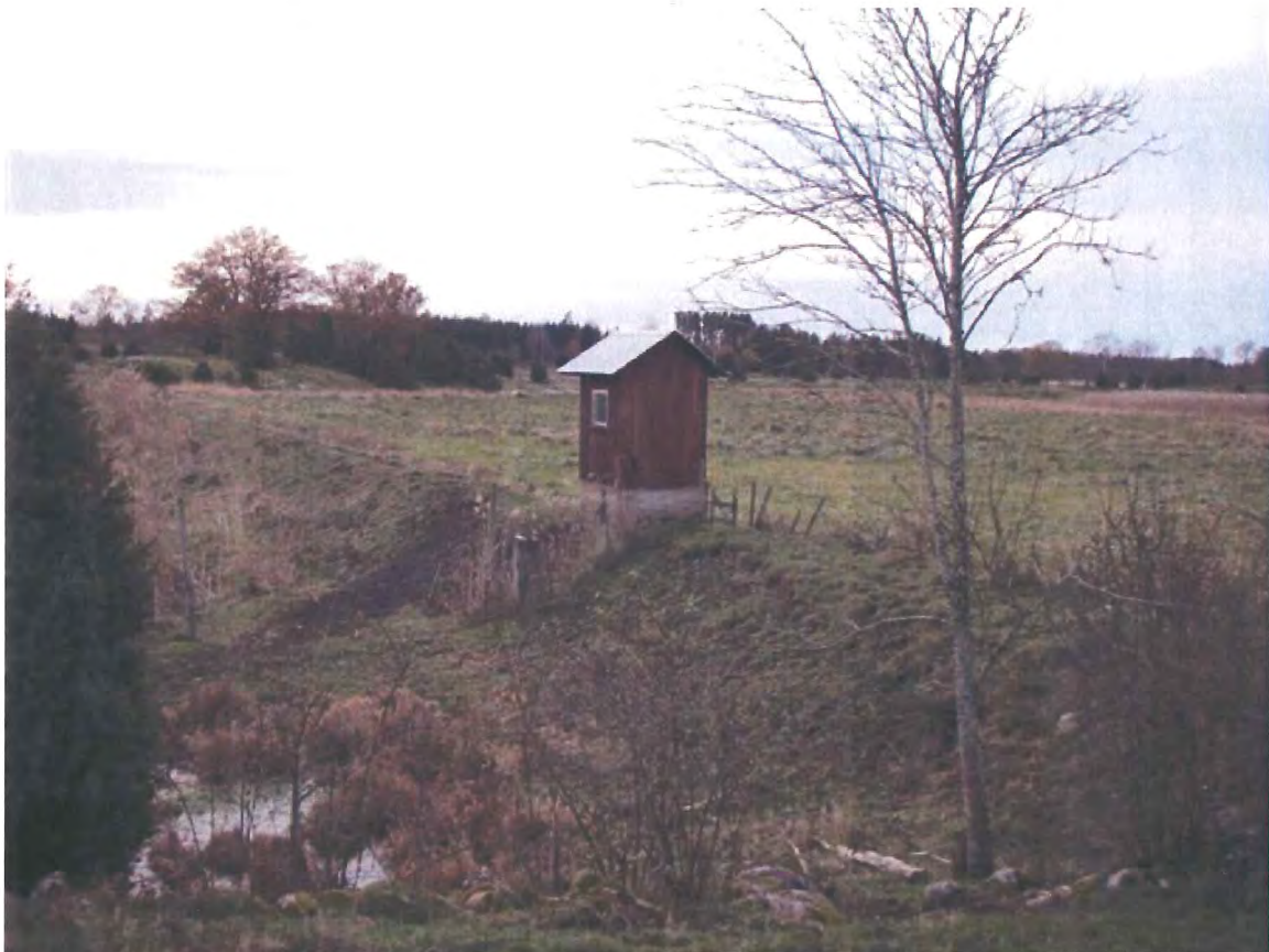
Photo 1. Pump house at the Skrukeby embankment.
