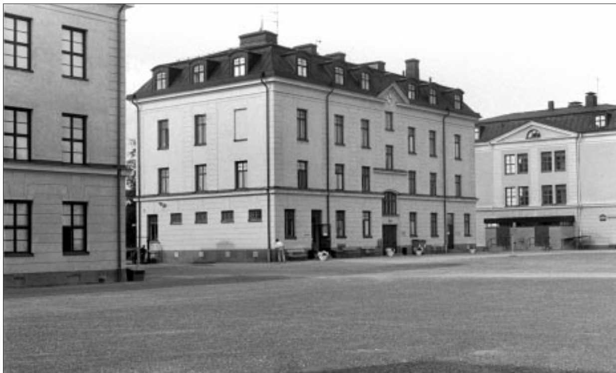
Kanslihus, Bodens garnison, regemente ing. 3 (1996).
