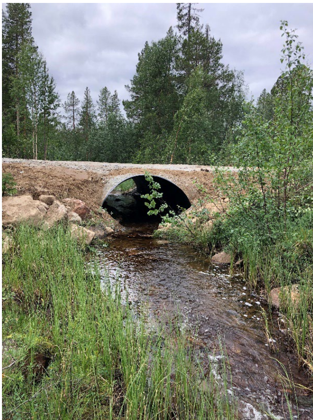
Figure 14. The photos are taken before and after remediation of migration barrier object 5. The old culvert was too narrow and the lack of bottom substrate didn't offer any resting size for fish. After remediation the water stream is wider. Inside the arch there is now the presence of bottom substrate together with bigger stones. Photo: County Administration Board.
