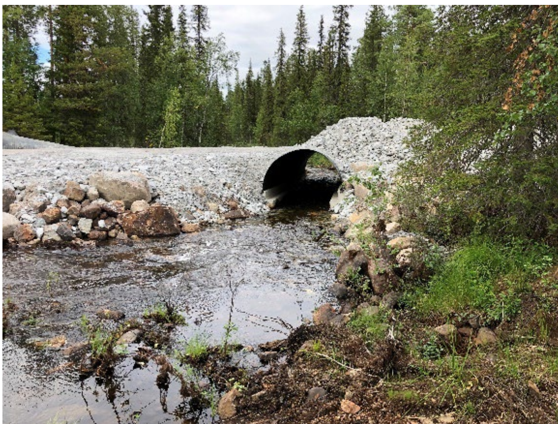
Figure 11. The photos are taken before and after remediation of migration barrier, object 2. A side channel to Pärälven river was reopened in the inlet and the increased waterflow required a wider bridge adapted to high water velocities and to avoid a too steep incline. Photo: County Administration Board.
