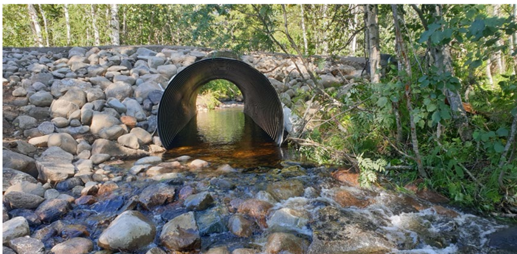
Figure 64. Sihtunajoki culvert after changing. A rapid was also built below to slow down the water flow and raise the water level in the road culvert. Photo: Lapland ELY-centres.
