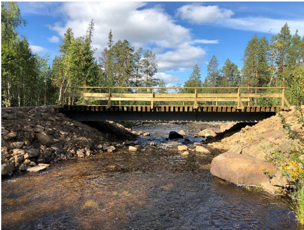
Figure 15. The photos are taken before and after remediation of migration barrier object 6. Before the remediation the bridge was too narrow, and it created a too high water velocity. After remediation the water velocity has decreased, the stream has regained its width and under the bridge there is now bottom substrate in different sizes. Photo: County Administration Board.
