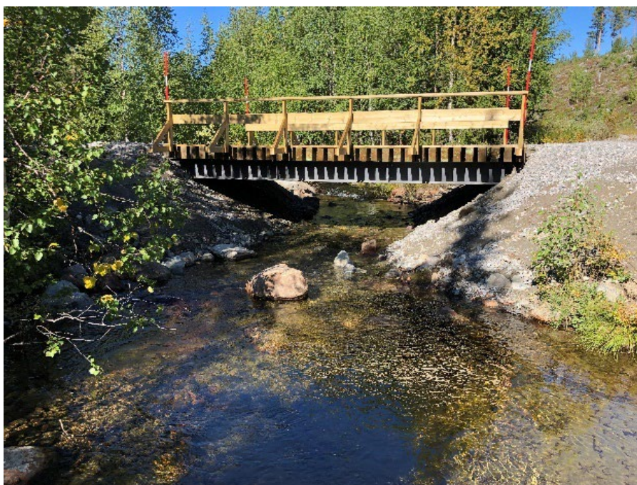
Figure 10. The photos are taken before and after remediation of migration barrier, object 1. Two culverts which both created a drop at the outlet. The culverts were also lacking bottom substrate. The long culverts have been replaced with a bridge so that the water stream can regain its original width and now also have bottom substrate mixed with bigger stones. Photo: County Administration Board.
