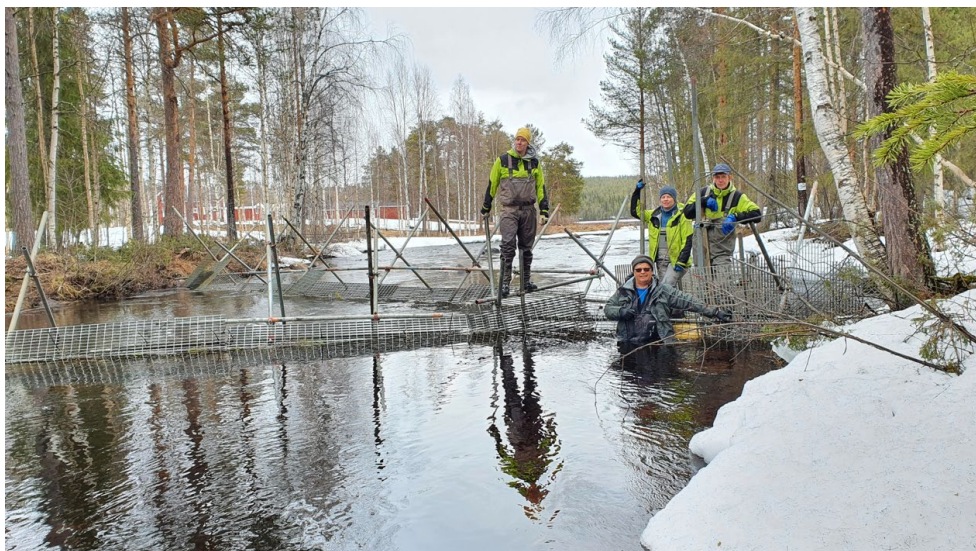
Figure 49. Installation of the fish counter in Linabäcken 2021. Photo: Administrative County Board in Norrbotten.
