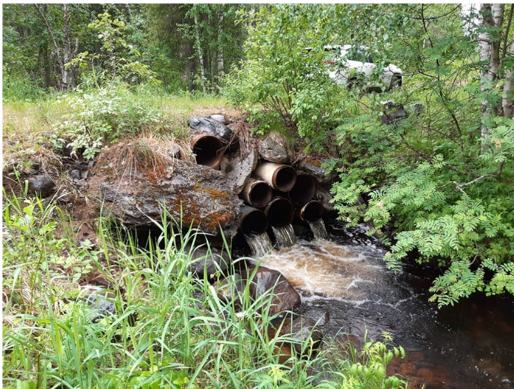
Figure 63. Sihtunajoki's seven-pipe culvert structure viewed from the downstream direction before culvert replacement. Photo: Timo Lettijeffer, Lapland ELY-centres.
