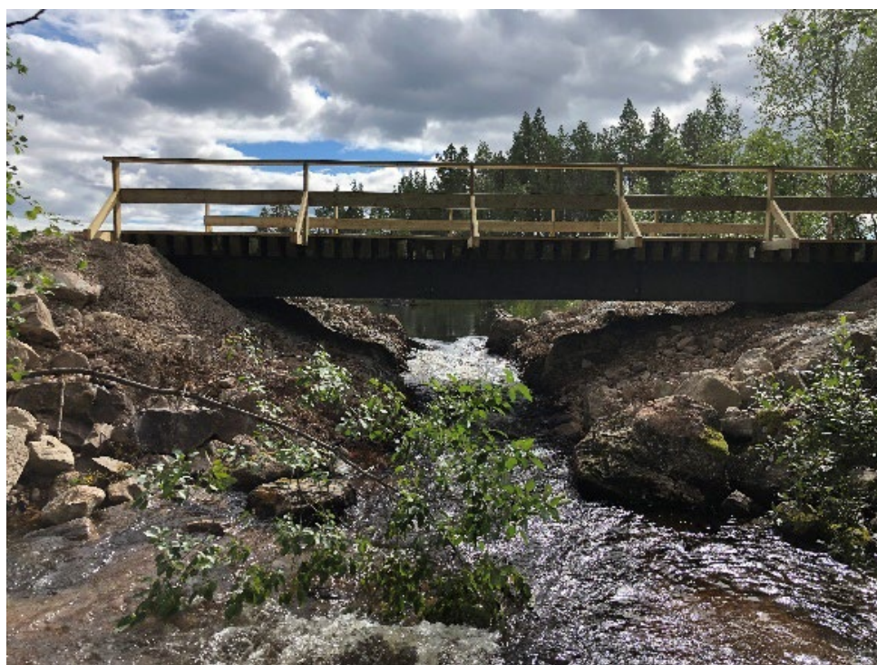
Figure 13. The photos are taken before and after remediation of migration barrier object 4. The old bridge had narrowed the water stream significantly. After the new bridge has been installed the water stream is wider. Photo: County Administration Board.
