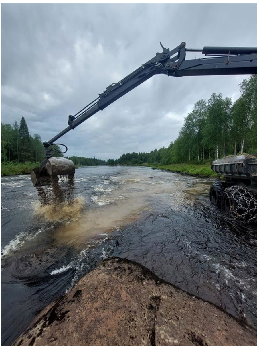
Figure 58. A forestry tractor laying spawning gravel in the Vikaköngäs rapid water sections. Photo: Antero Mölläri, Metsähallitus
