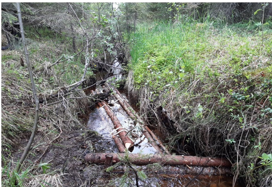
Figure 62. At the bottom dam, the water level in the shallow ditch was raised so that the tree trunk bundles stay below the water level. Photo: Reeta Peteri, Lapland ELY-centres.
