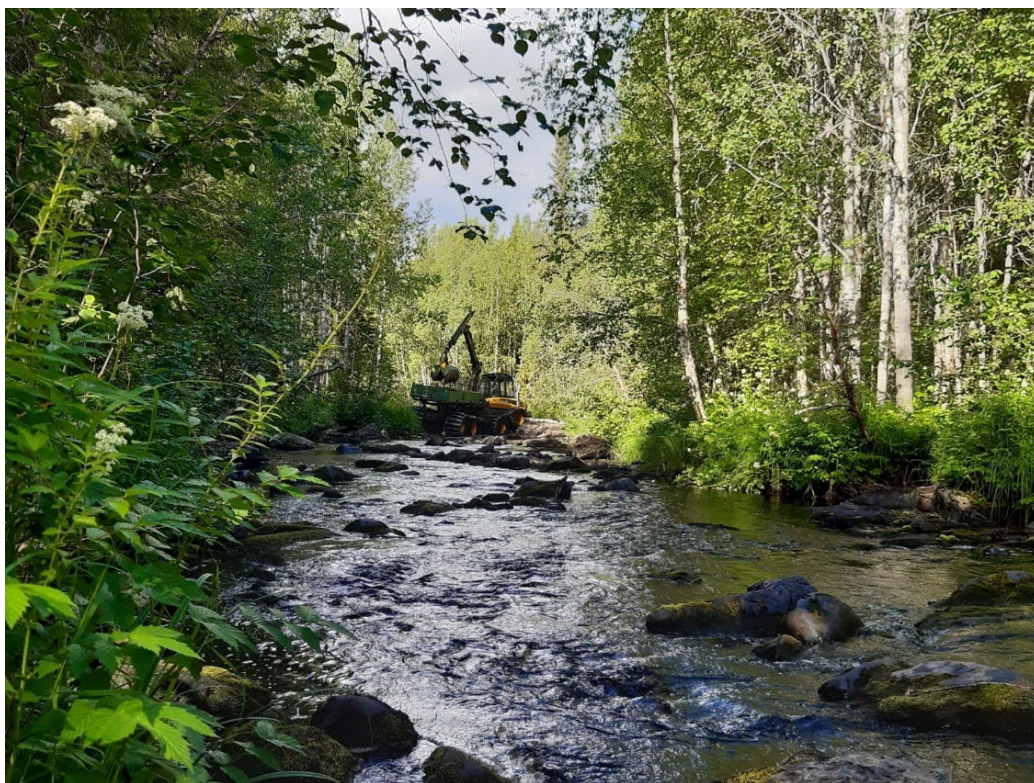
Figure 65. Laying of spawning gravel with a forest tractor in Ropsajoki in the summer of 2022. Photo: Piia Sonkajärvi, Lapland ELY-centres.
