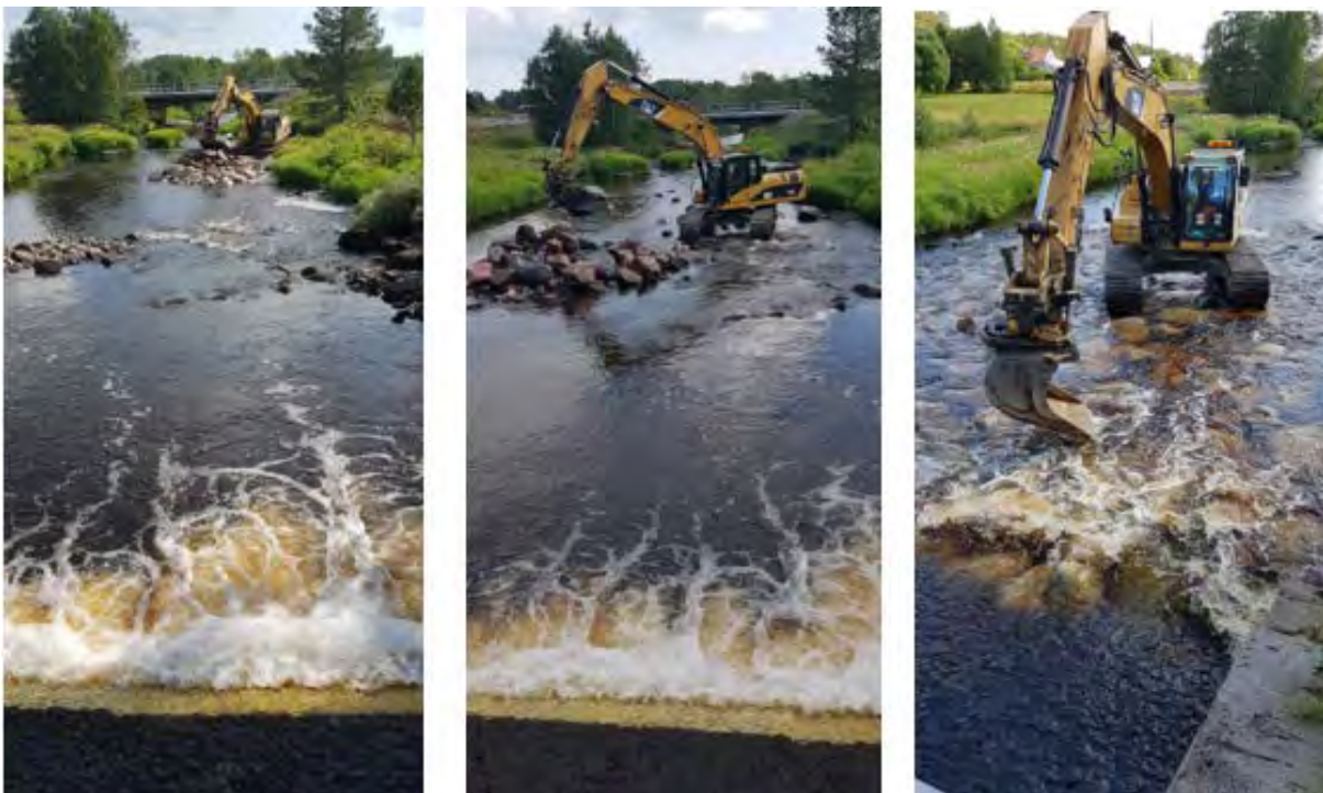
Figure 4.17. Arranging boulders and rocks at Ale Kvarn in the Alån river.
