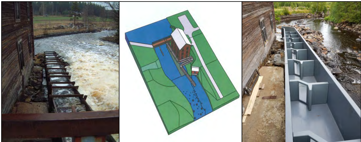
Figure 4.4. The old fishway to the left and the new fishway to the right, manufactured in composite with slot openings 2018.
