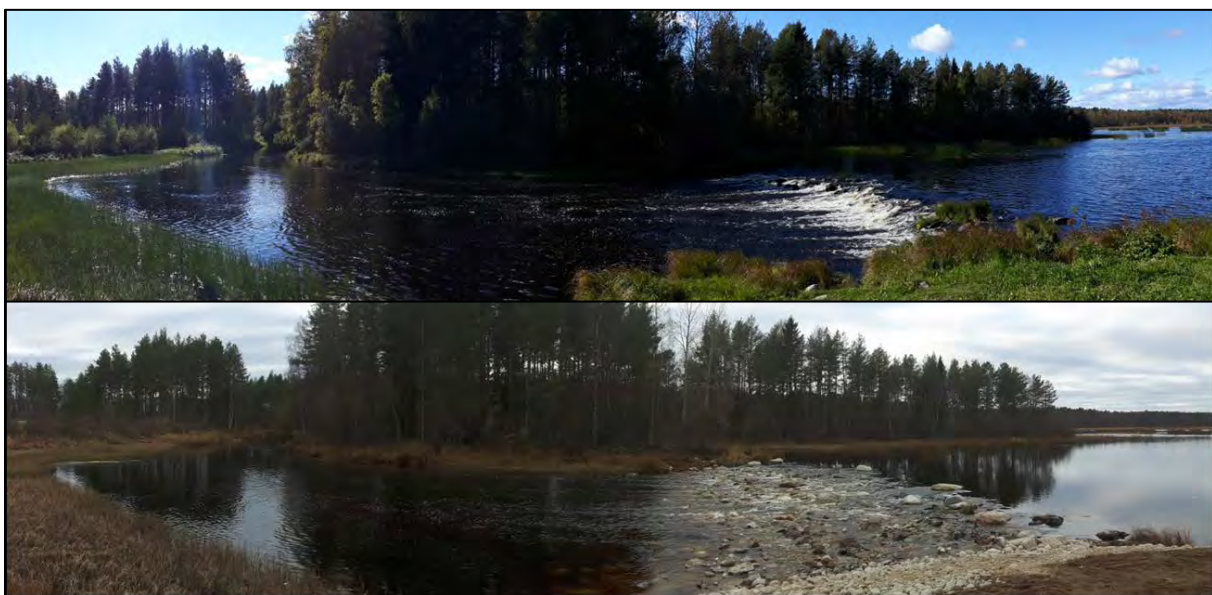
Figure 4.3. Porsnäsdammen before (upper photo) and after (lower photo) remedial work in 2016.
