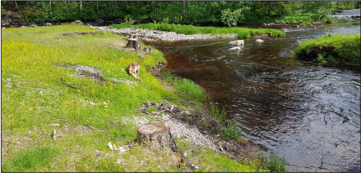
Figure 4.26. Transport route of the excavator and dumper truck at Selets Bruk with barely visible rutting on the slope between the two nearest tree trunks. The side channel is on the right of the picture and the main channel at the top of the picture.
