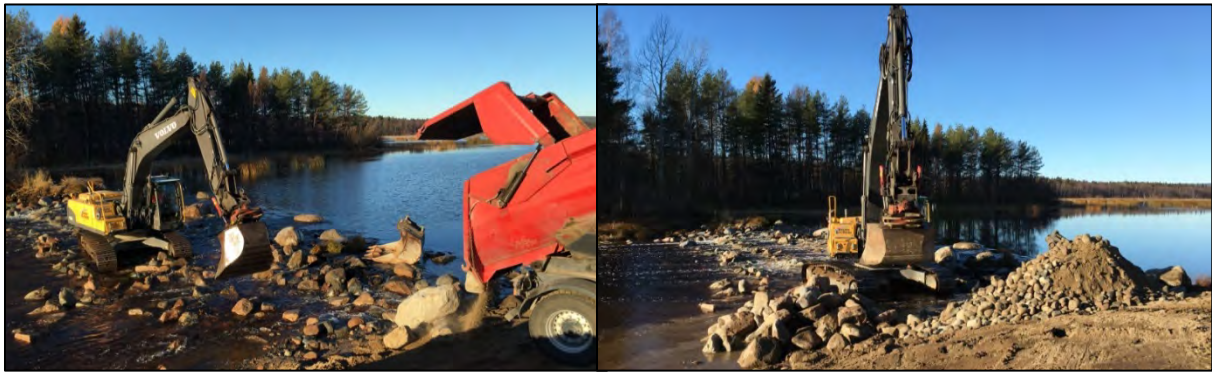
Figure 4.2. Transport and arranging the rock using an excavator.
