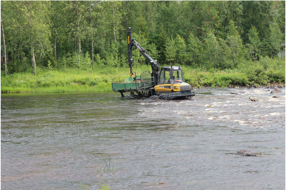
Figure 6. Transport of spawning gravel to the restoration site at Harskukoski rapids, 2017.
