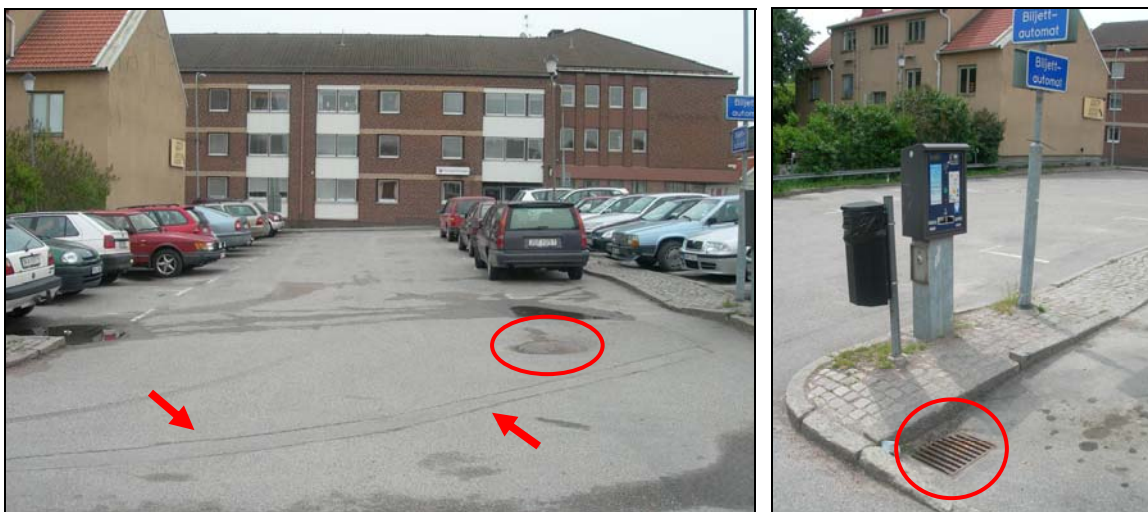
Figure 3.3.3: Trench intrusion in asphalt surface in the south-western part of survey site Äkroken (upper part) and manhole cover (photo left). Indication for sewer pipes in the subsurface can be seen as well in the right photo.
