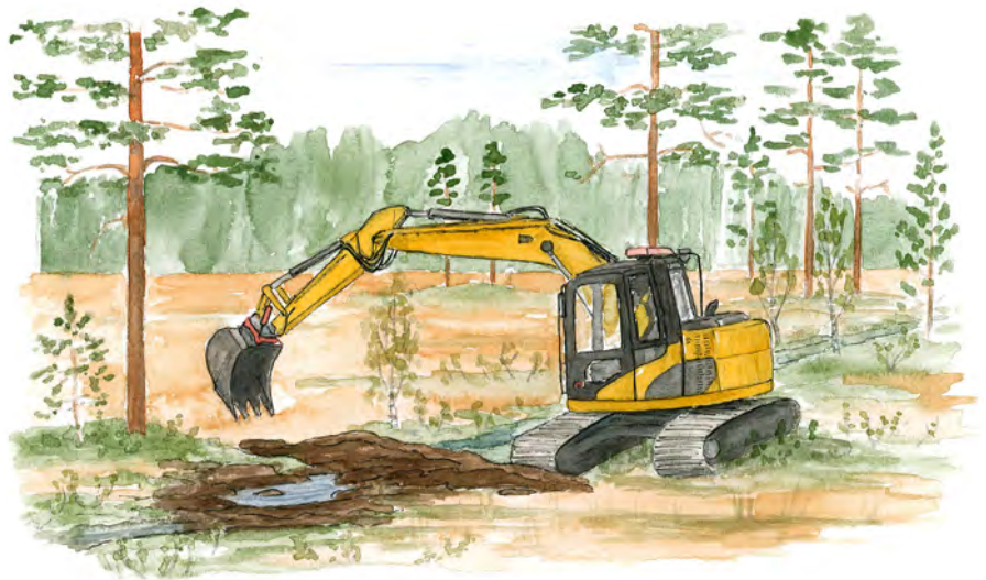
To the left: Excavator on a mat of trunks building a dam.
