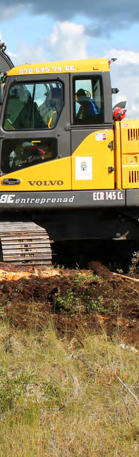
To the left: Excavator on a mat of trunks building a dam.
