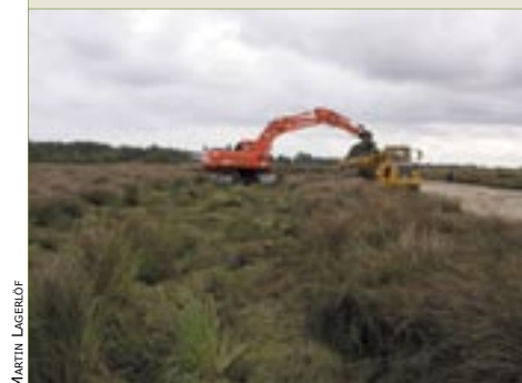
As part of the restoration, sediment and peat were removed by an excavator and dumper trucks
