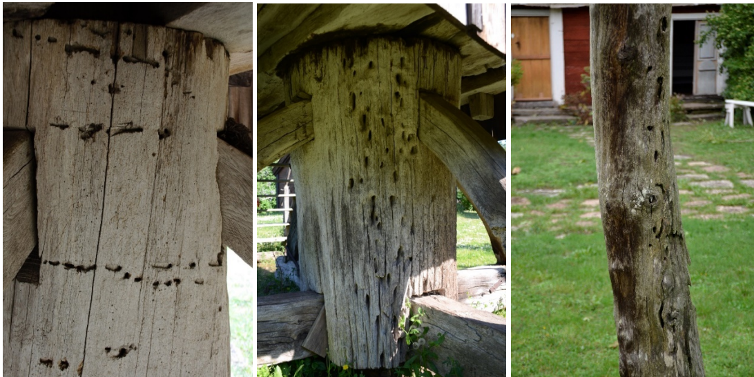
Two of the eighteenth-century mill stubs and a wellhead in Himmelsberga with (probable) larger wood-boring insect damage.
