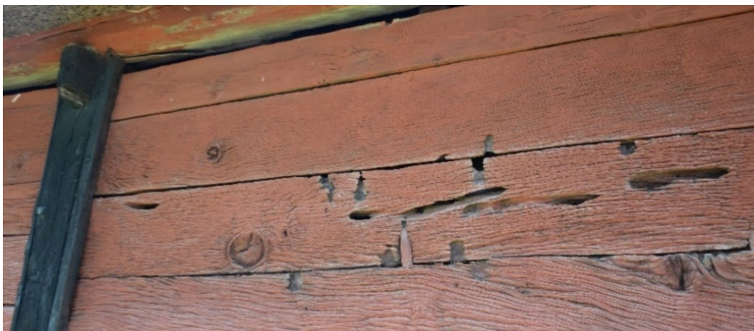
A millstone plank from the millstone shed at Lindbergsgården in Algutsrum with probable gnagspår of larger wood-boring insect.
