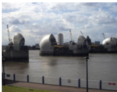
Figur 116. Thames barrier – London, UK.
